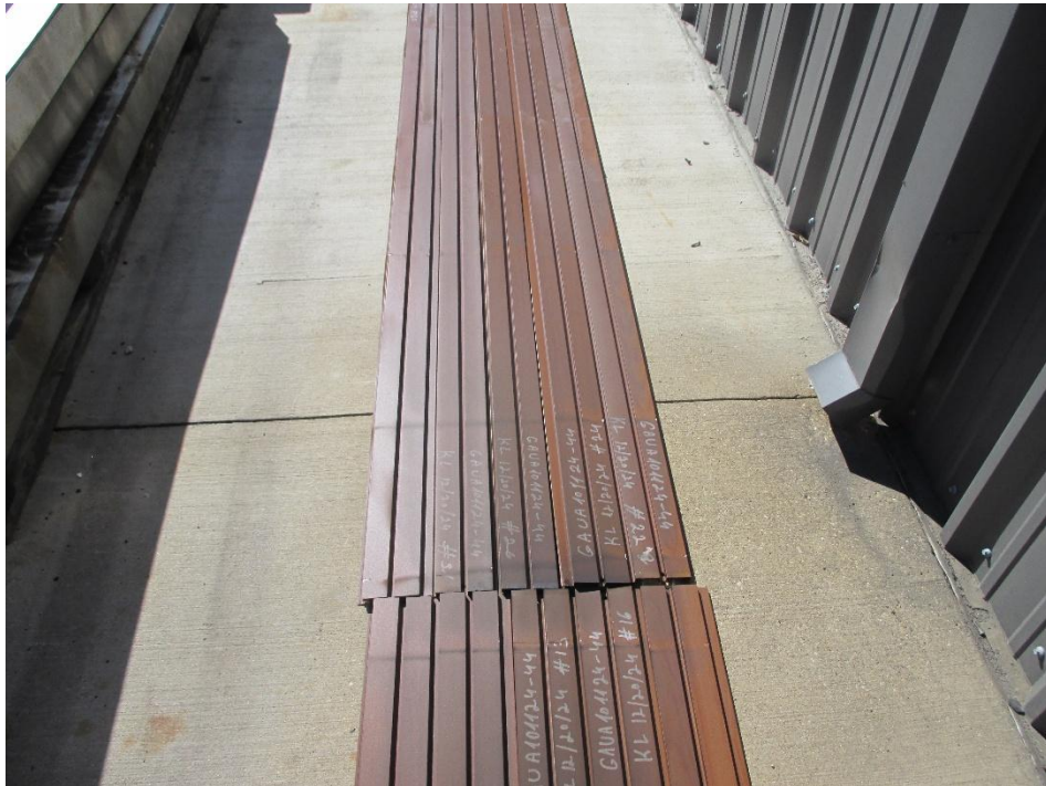
Photo No.6 Post-Test Exposed Side (Continued)
